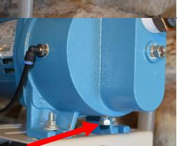
Unscrew the tap at the bottom of the pump.
